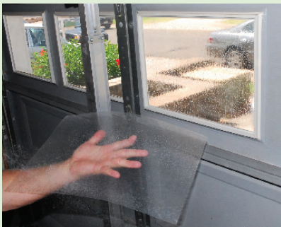
Figure 4-15. Laminated film comes in various thicknesses and strengths. Here the film is applied to an existing window before it is bead-locked to the frame with silicone structural sealant.
