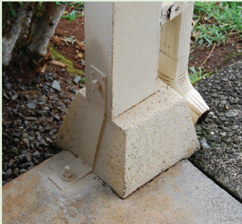
Figure 4-6. In some retrofit examples, it is possible to tie a portion of the house to the foundation. Here, a metal strap connects the vertical post to the foundation, which finishes the continuous load path connection from roof to the foundation. Photo courtesy of Hurricane Protection Services.
