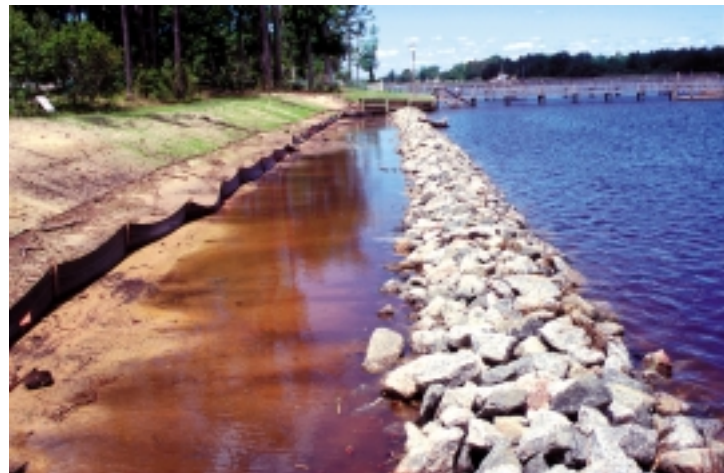
Same shoreline after regrading of eroding banks and stabilization with stone sill.
