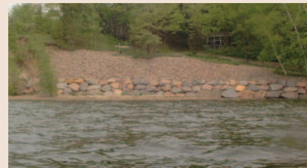
A stone riprap revetment combines smaller placed rocks on the face of the bank and larger rocks to help stabilize the toe of the bank near the waterline.
