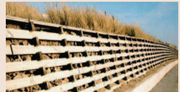
Timber crib walls, typically constructed using Douglas fir, are not commonly built on Lake Champlain's shores; they could be adapted as seawalls.
